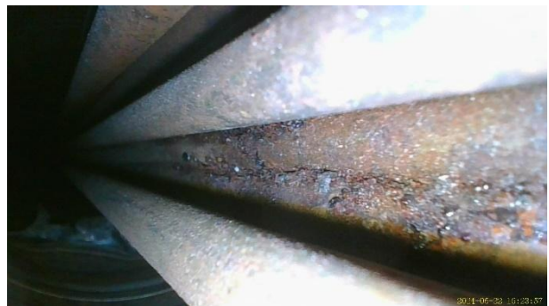
Figure 55 Opening 3N – Images of Duct 31N; Views of spreading cables entering the anchor, confirming void status
