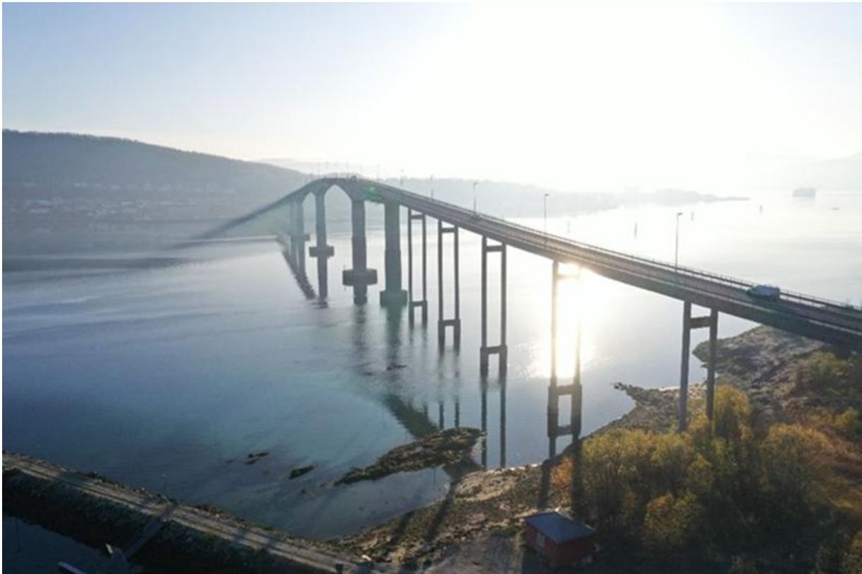
Figure 38 Overview of Gisund Bridge
