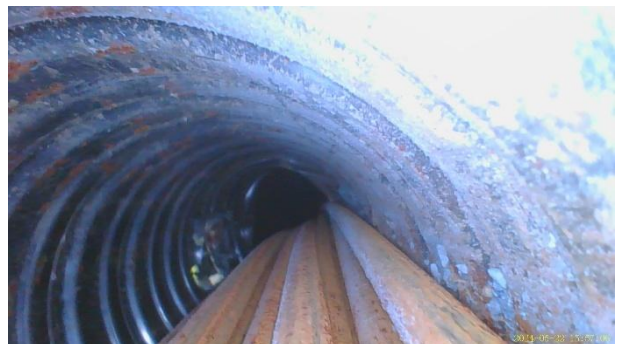
Figure 54 Opening 2N – Images of Duct 31N; Photos showing tape around strands and empty duct interior
