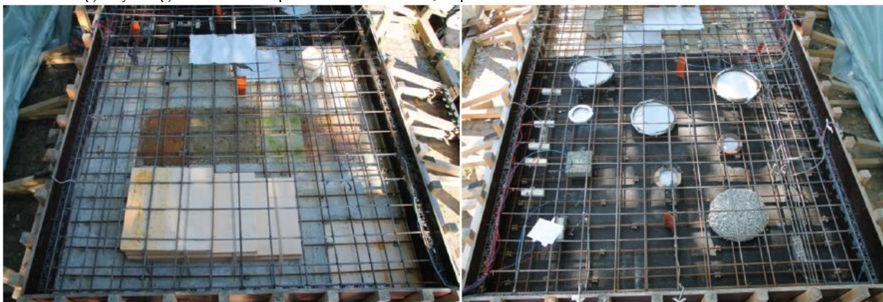
Figure 12 Photos of the mock-up before concreting
