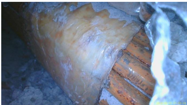
Figure 54 Opening 2N – Images of Duct 31N; Photos showing tape around strands and empty duct interior
