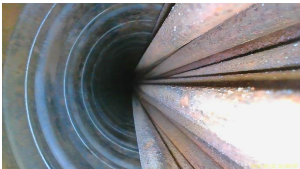
Figure 55 Opening 3N – Images of Duct 31N; Views of spreading cables entering the anchor, confirming void status
