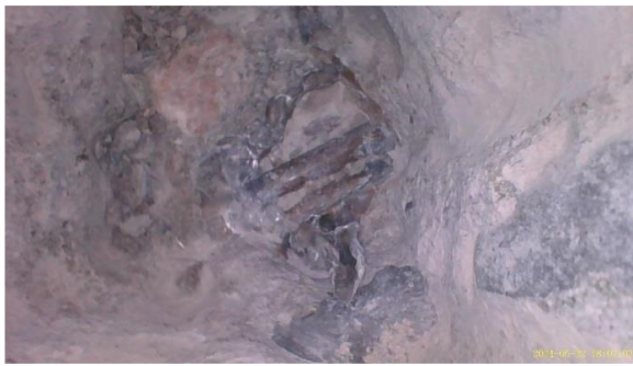
Figure 57 Opening 7N - Image of duct 34 with grout
