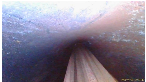
Figure 53 Opening 1N – Images from Duct 31N near anchor in X13; Left: View toward the anchor; right: Exposed strands
