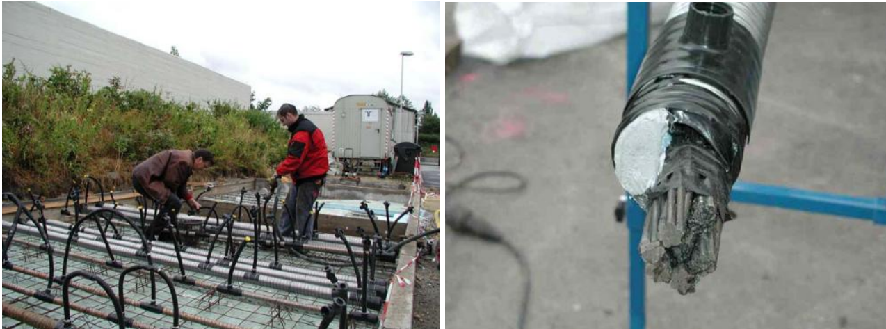
Figure 11 Left: Tendons being installed in the Large Concrete Slab (LCS) prior to grouting. Right: Close-up of a tendon duct containing prestressing strands with an intentionally created artificial void, prepared before placement in the slab
