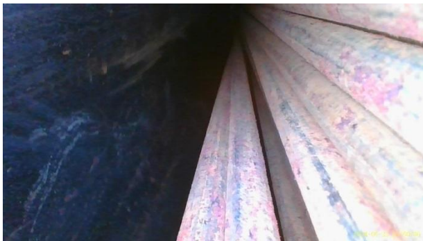
Figure 53 Opening 1N – Images from Duct 31N near anchor in X13; Left: View toward the anchor; right: Exposed strands
